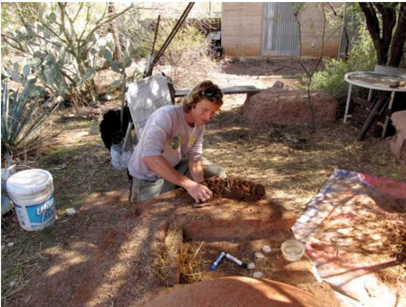
Above: The beginning of a cob wall made with clay soil found on site
