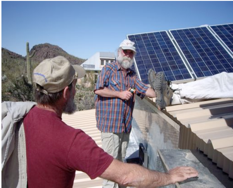
Above: Solar Grid-Tie installation on Barn, SEI Course, February 2007
