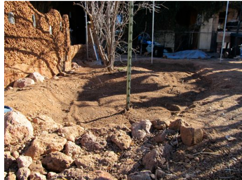
Above: Waterharvesting swale around a pomegranate tree
