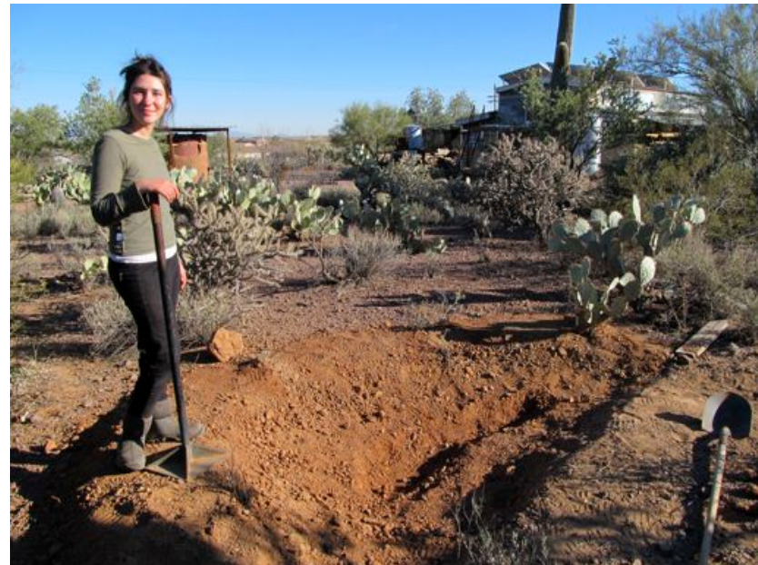
Above: Intern digging water harvesting swale
