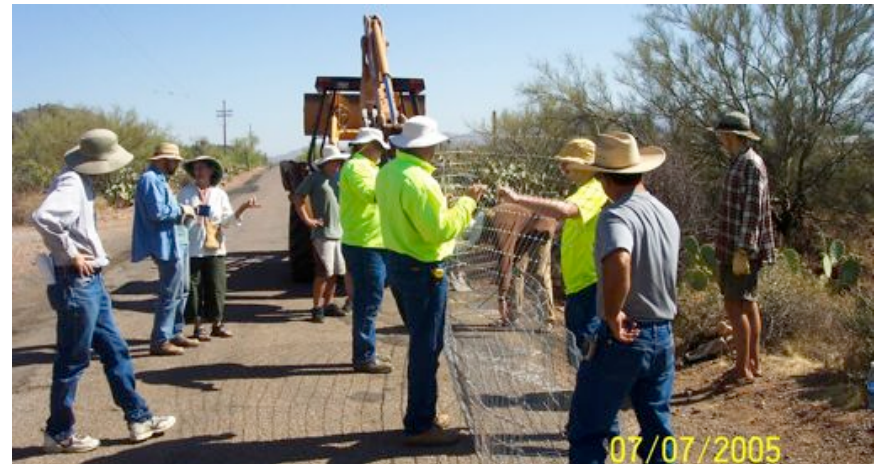
Workshop team prepares to install gabion.
