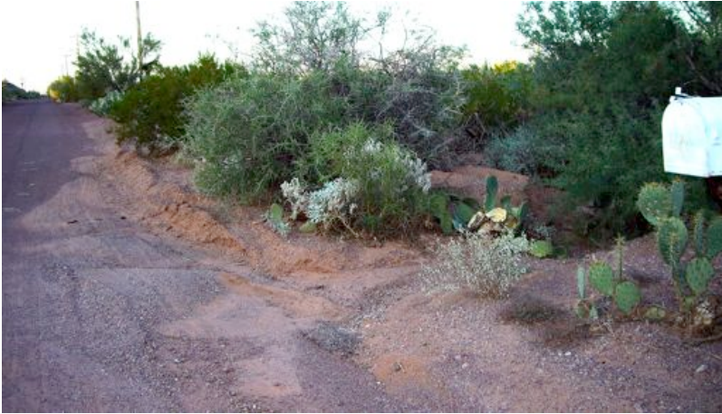
Waterborne soils from upstream erosion are deposited on Scenic Drive
