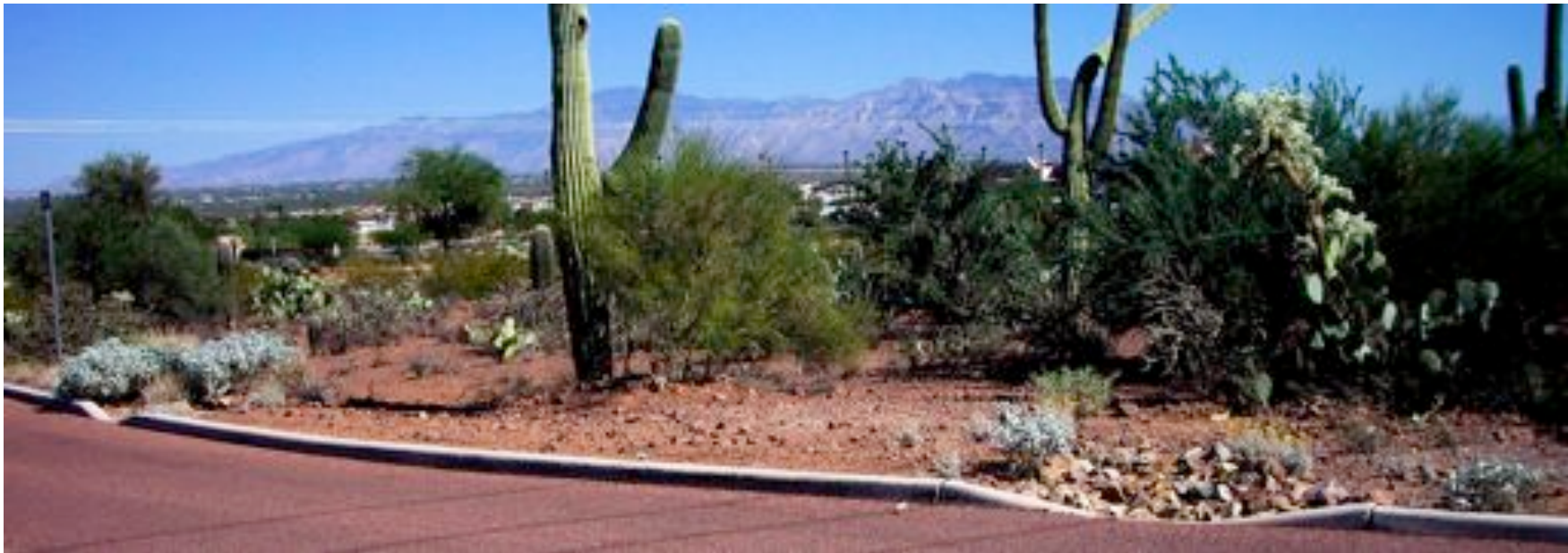
North end of Scenic Drive showing curb cuts for harvesting rainwater. Town of Marana Road Realignment.
