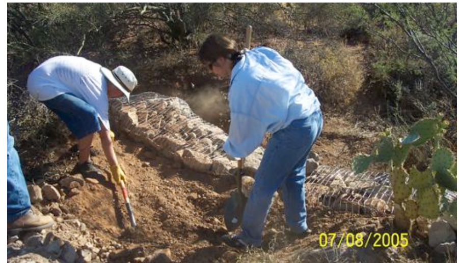
Neighbors and Town staff complete gabion earthworks.
